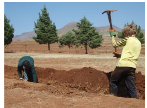
Digging the trench
